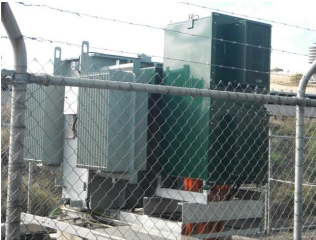
Fig 27 – 2MVA Forced Cooled Module 2011
