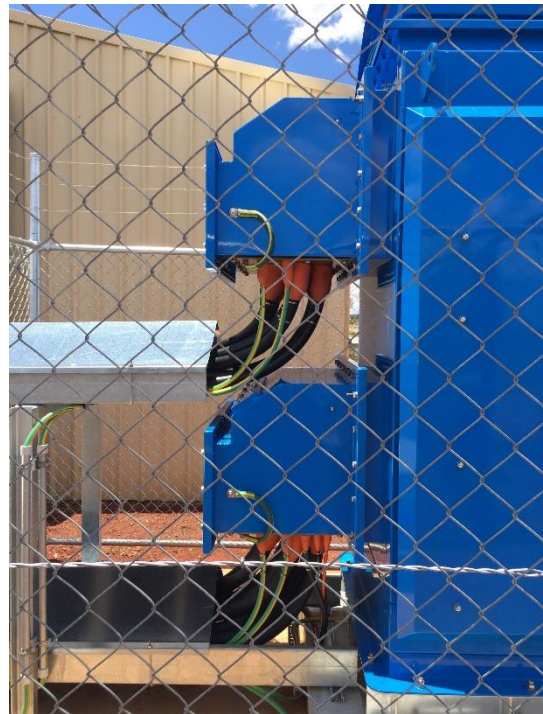
Figure 9 – Typical 6 x 630mm 2 / Phase Installation
