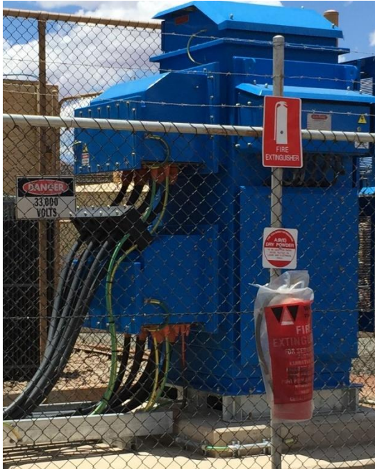
Figure 10 – Typical 3 x 500mm 2 / Phase Installation
